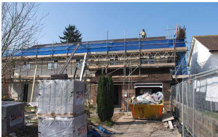
Retrofitted homes with external wall insulation, high efficiency heating and glazing, and solar panels on the roof. Radian - 2010 Ashden
