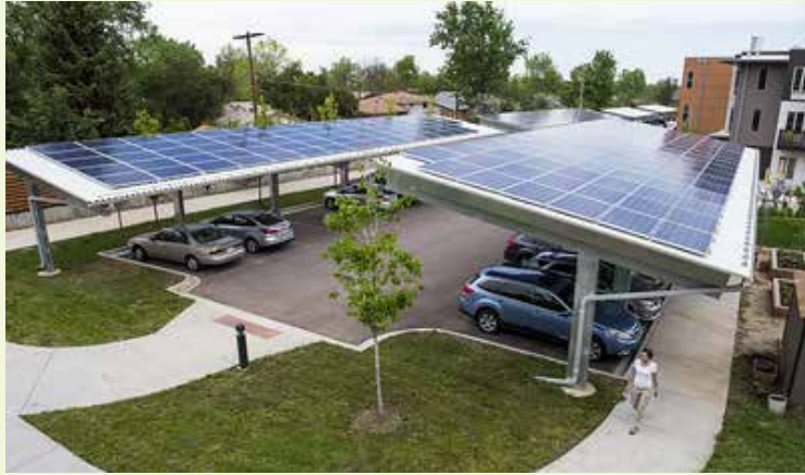
Solar Parking Lot. Photo: Dennis Schroeder
