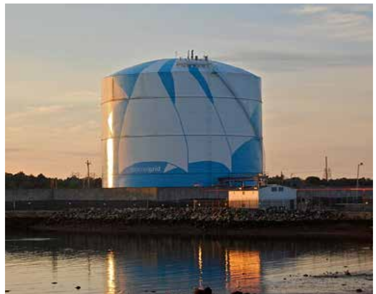
A liquefied natural gas storage facility in Massachusetts commons.wikimedia.org/wiki/File:National_Grid_LNG_Tank.jpg
